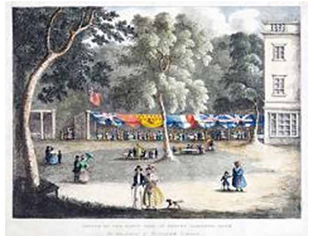
Figure 16 Sydney Gardens and the entrance from (New) Sydney Place, c. 1840
